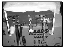
6. Assemble and tighten the following parts to make the *heating supply and cold water mains inlet* as shown below. Attach (c) the <sup>3</sup>/<sub>4</sub> copper 90° to (l) the red ball valve. Add (i) the silver 90° to (l). Attach (k) the red handled mixing valve next. Now finish with (e) copper 90° and (j) the <sup>1</sup>/<sub>2</sub> copper 90°. Ensure all fittings are tight and aligned as shown.
