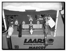
6. Connect and tighten part (a) ½ black handled ball valve to part (e) ½ x 90° copper elbow. Install assembly to (4) cold water mains inlet.
