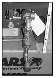
5. Attach part **(f)** yellow handled gas ball valve w/elbow to the gas inlet **(3)**. Make sure to tighten both the elbow to the ball valve as well as the gas inlet connection.
