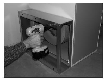
Skuttle's pre-punched holes make installation of the Air Cleaner cabinet faster and easier.
