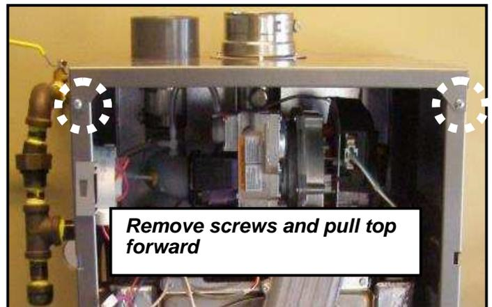
**Figure 4A: Typical Burner Door Assembly:**
