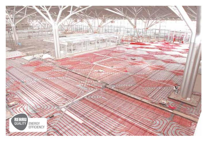
RADIANT HEATING AND SNOW AND ICE MELTING SYSTEMS
